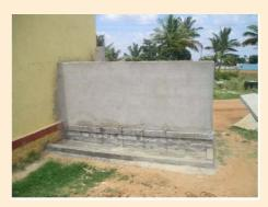
Water taps outlet system and cemented area below the tap for letting wastewater disposal
